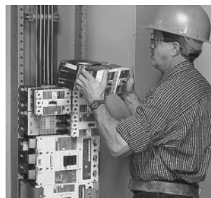
Panelboard Installation
