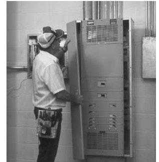
The Three-Piece Trim for Larger Power Distribution Panelboards Provides for Easy Handling and Installation
